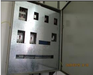
Photo of the inside of the main production hall Electronic box with inner cover.JPG
