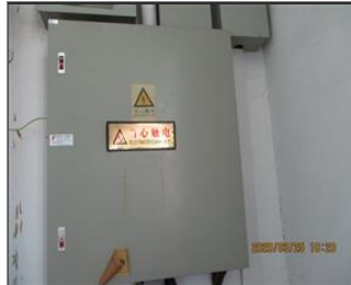
Photo of the inside of the main production hall Electronic box with warning sign.JPG
