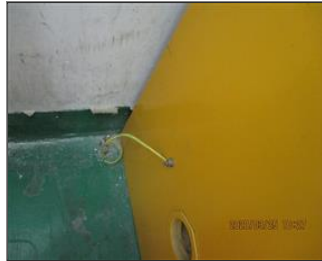
Photo of chemical storage room (if applicable) Explosion proof cabinet is grounded .JPG
