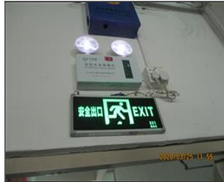
Photo of fire safety equipment Fire emergency lighting.JPG
