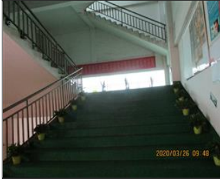
Photo of fire safety equipment Fire stairs.JPG
