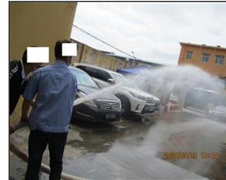
Photo of fire safety equipment Fire hydranting testing.JPG
