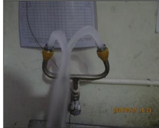
Photo first aid facilities Eye washing facilities.JPG
